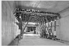
Tunnel Formwork
