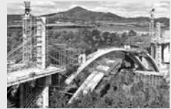
Bridge Formwork
